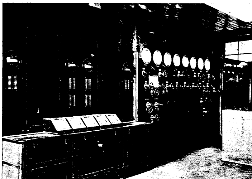
Fig. 19. Control post and measuring instruments.
